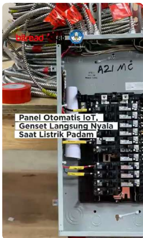
Video 1: Panel otomatis IoT, genset otomatis nyala saat listrik padam.
