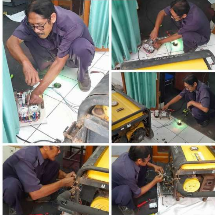
Gambar 2: Uji coba Panel ATS/AMF
